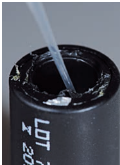
16. use SHOTBOND® to optimize bonding
